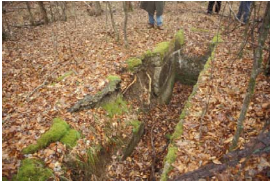
Compromised dipping vat
