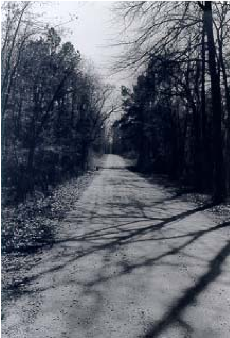
The Dollarway Road near Redfield in Jefferson County. AHPP photo.
