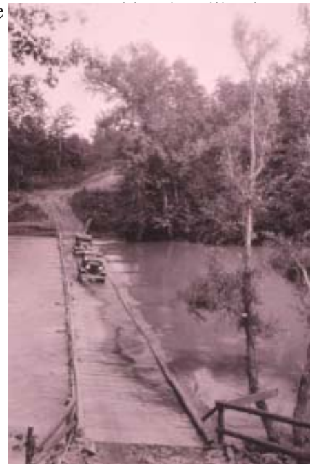
Travelers brave a flooded bridge on the Fourche River. Ouachita National Forest photo.
